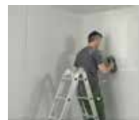
Smooth finely with spatula two to three times and polish transitions.
