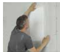
Stretch out glass fiber fabric, smooth down and leave to dry.
