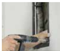
Insert frame and secure feet.
