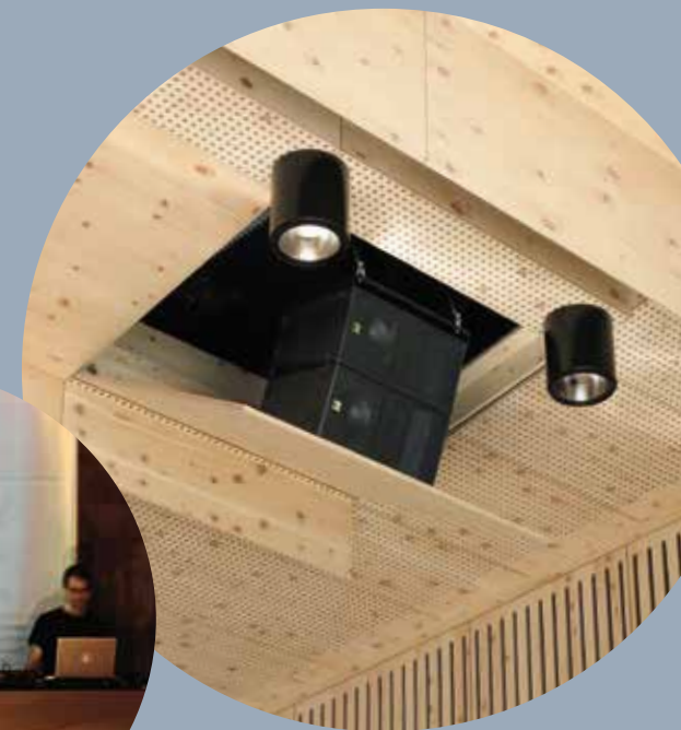
Freilichtbühne St. Martin in Passeier South Tyrol PA system with line arrays
